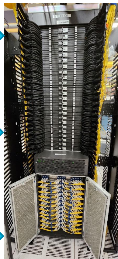
8812 Front w/ Cable Mgmt 1728 x 100Gb ports
